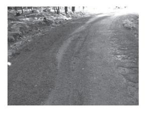
If you end up after a few passes looking like this, you are doing it right. Notice that the edge material is filling the rut and the higher center is just barely scraped. With practice, you will find the best combination of weighting, speed and angle to do the best job.
