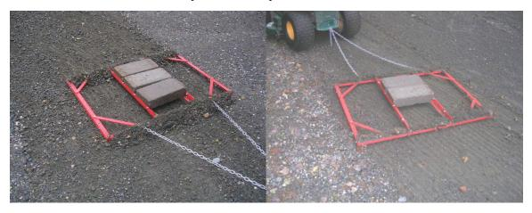
If you have an A shape crown with just some ruts and bumps, drive up and down each edge separately fully loaded first.
