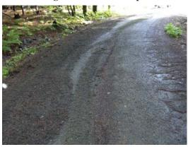
If you end up looking like this, you are doing it right. Notice that the edge material is filling the rut and the higher center is just barely scraped. With practice, you will find the best combination of weighting, speed and angle to do the best job.
